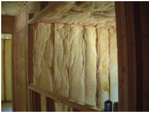
Rebuilding and insulating the train room to minimize sound
