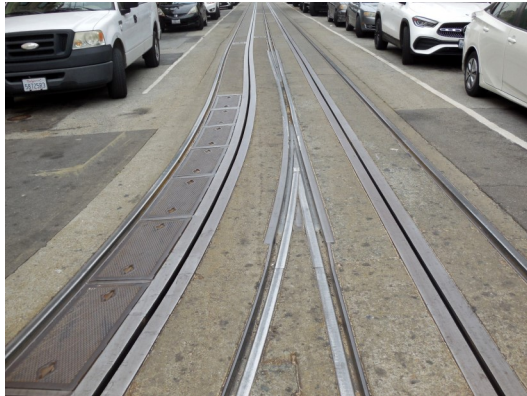
Two views of the split at the end of the gauntlet track. Above, looking downhill. Below, looking uphill.
