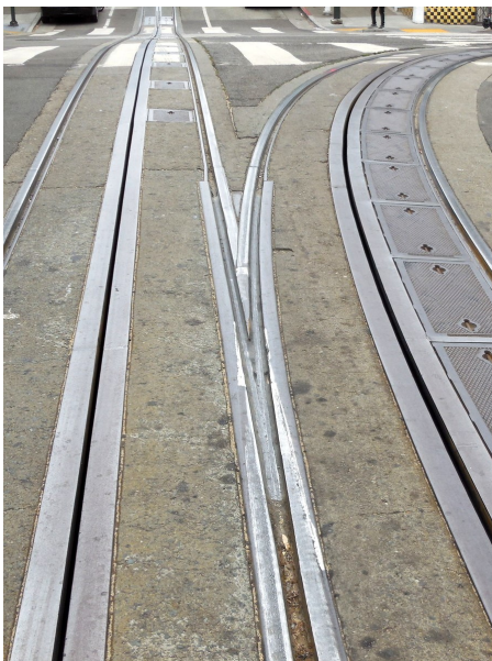
Two views of the split at the end of the gauntlet track. Above, looking downhill. Below, looking uphill.
