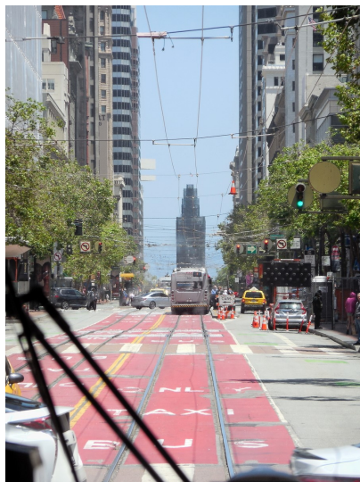
The Ferry Building clock tower is undergoing restoration and is shrouded in scaffolding and netting.
